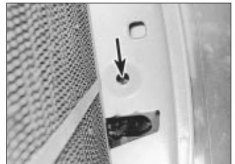
7.9 Access hole (arrowed) below bonnet lock
