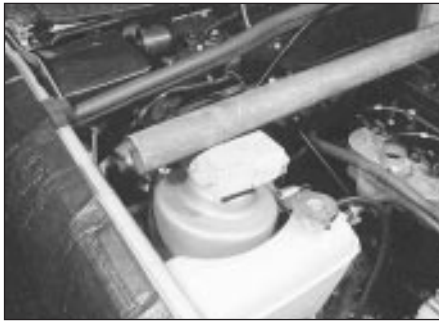
29.9a Make up wooden blocks to fit the front suspension turrets and support a metal bar . . .
