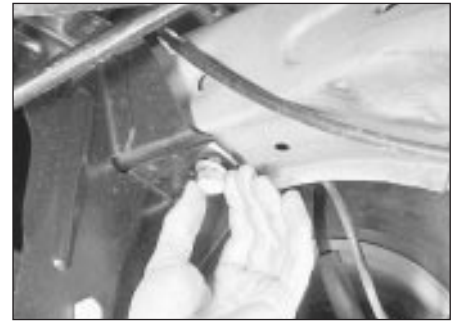
29.10 Unscrew the front crossmember securing bolts
